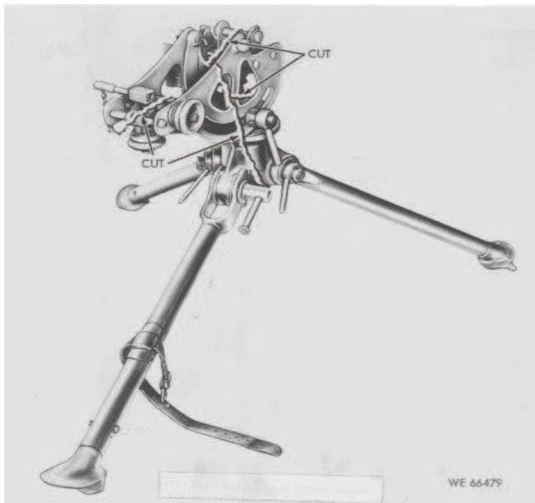
Figure 6. Machine Gun Tripod Mount
