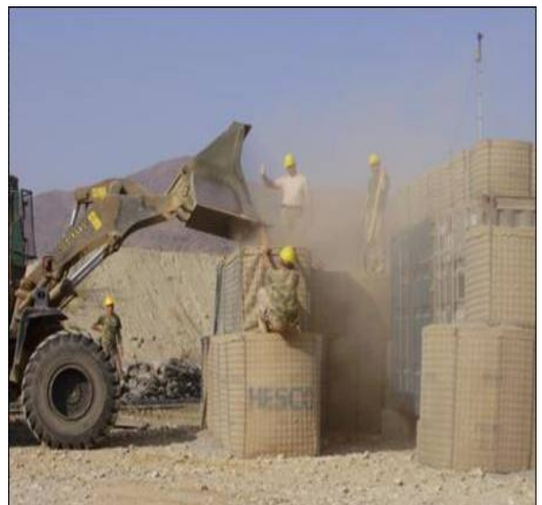
Loading HESCO with aggregates _ September 2009
