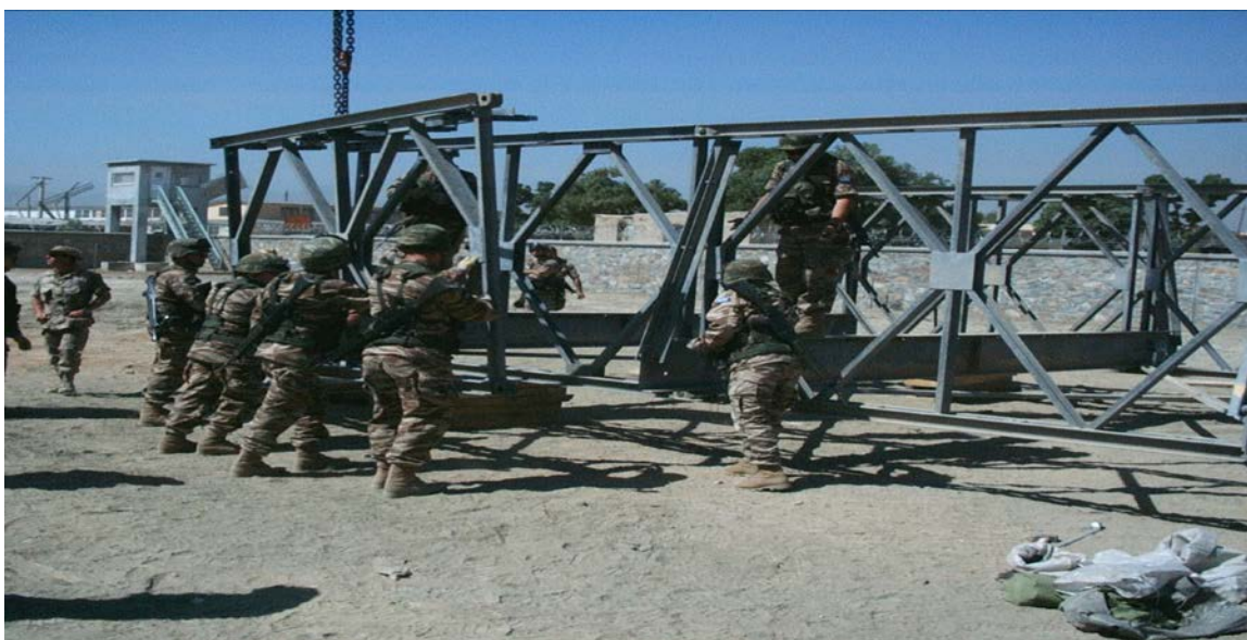
Constructing an MABEY – JOHNSON bridge_ May 2003
