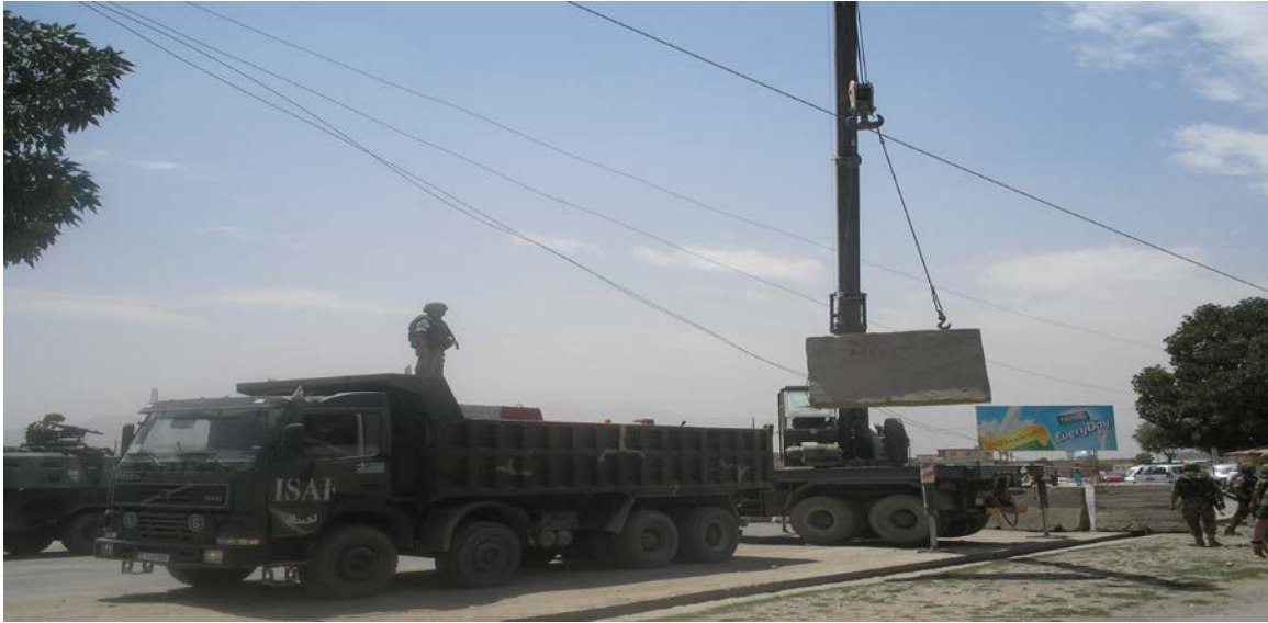
Transfer of NEW JERSEYS BLOCKS by a GRC dump truck with the assistance of an ITA crane_ May 2007
