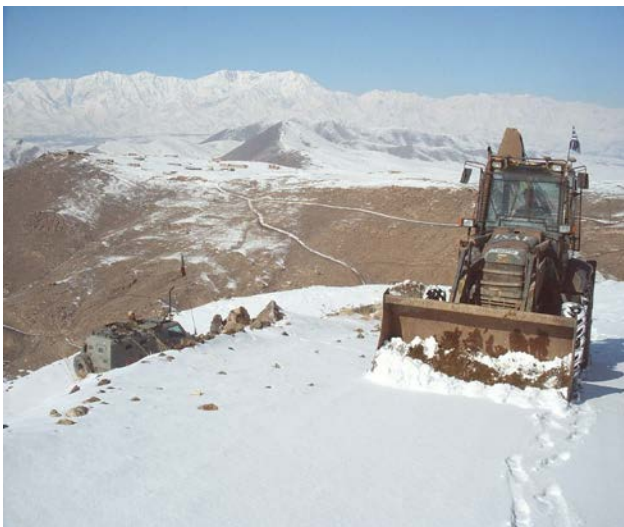
Snow clearing works at the RADAR HILL _ January 2005
