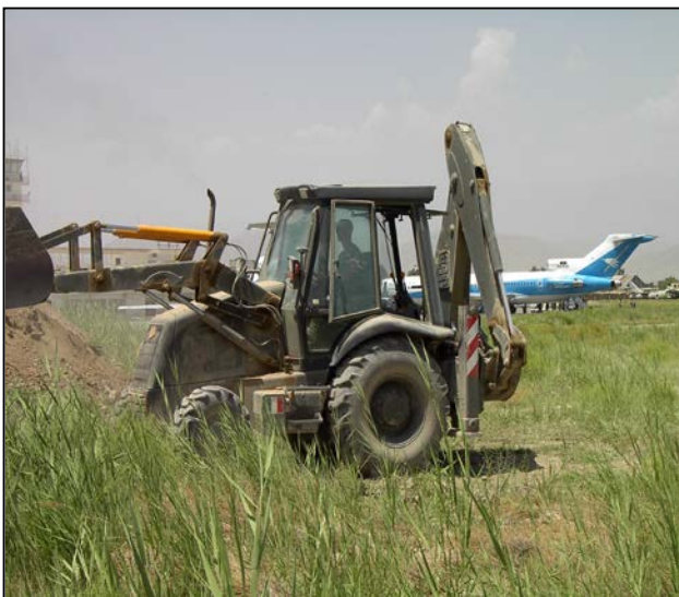
A back hoe loader working near by the KAIA runway_ July 2002
