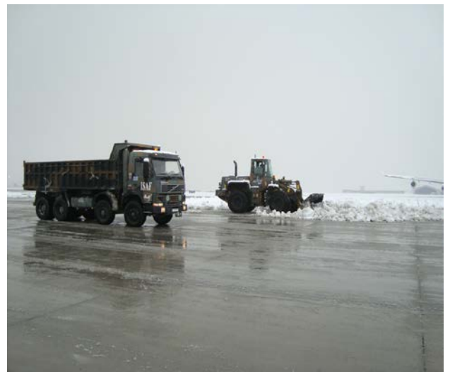
Snow clearing works at the KAIA runway _February 2010
