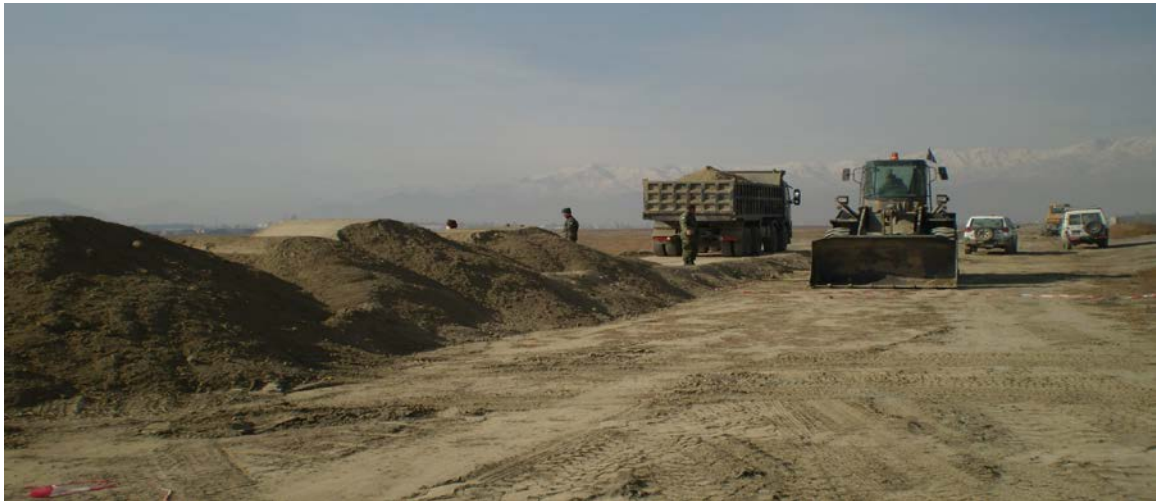
Construction of embankment at KAIA North _From November 2008 to March 2009
