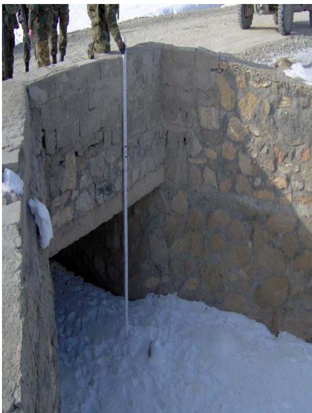
Engineer Recce _ March 2005
