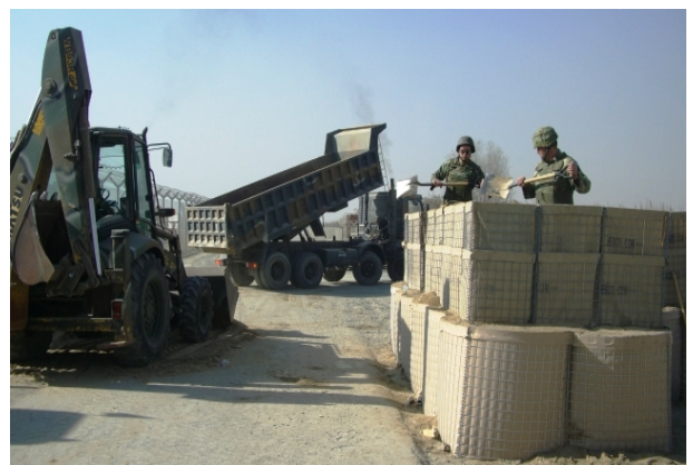
Construction of fortification positions and installation of HESCO bankers _December and January 2011
