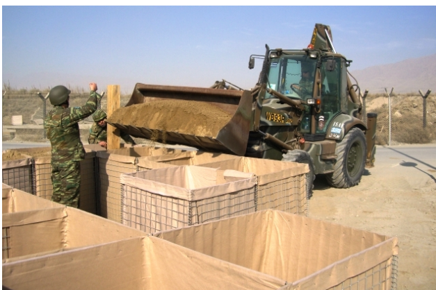
Construction of fortification positions and installation of HESCO bankers _December and January 2011
